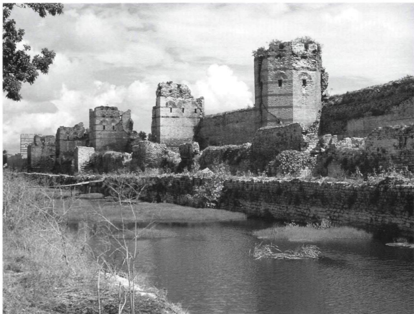
Towers and walls of the inner wall between the Golden Gate and the Belgrade Gate. The first tower is octagonal. Although damaged here, we can also clearly see the outer wall, the other small wall outside the outer walk, and the moat, here flooded. (Stephen Turnbull)
