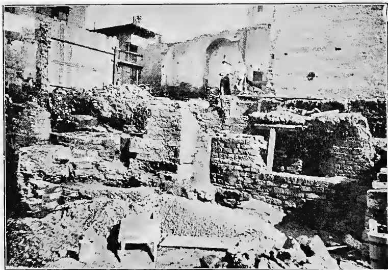
EXTERIOR VIEW OF CALIDARIUM AND FURNACE.
