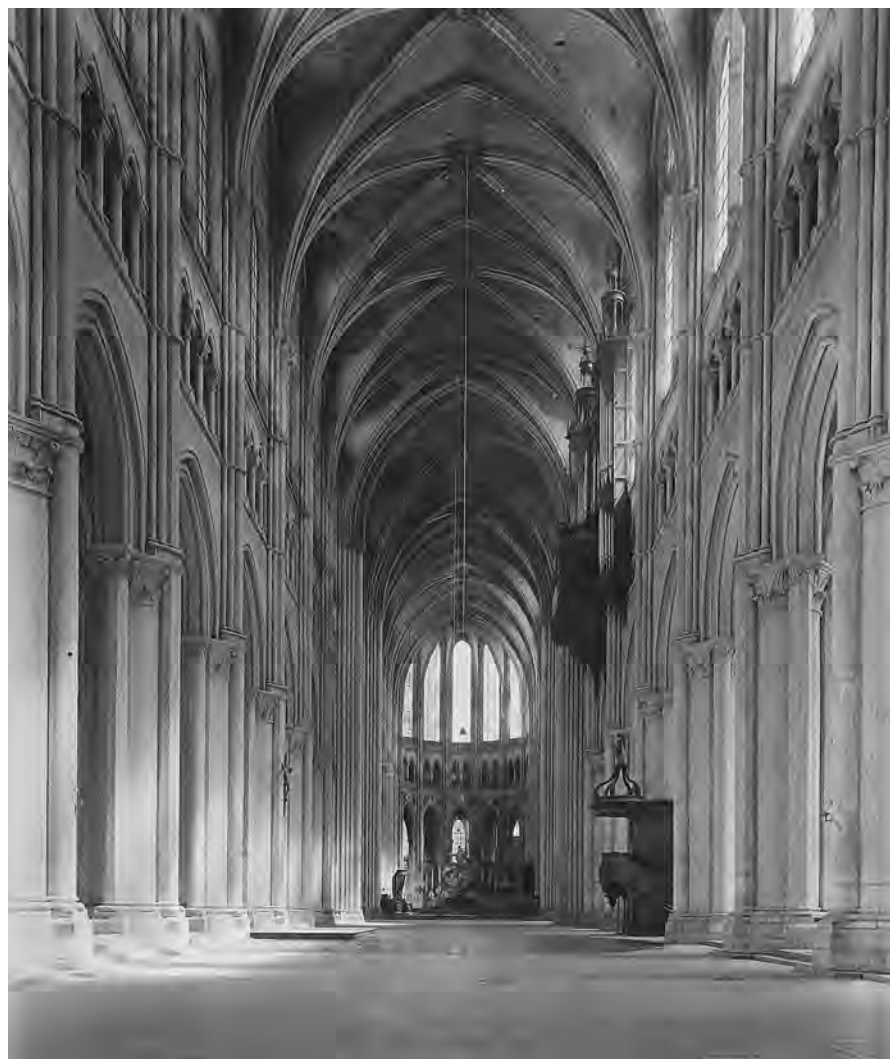
Plate 2 Chartres cathedral, nave, after 1194
