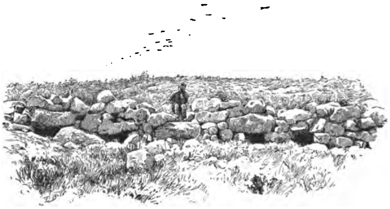
Fig. 8. Cyclopean Road, showing Drains
