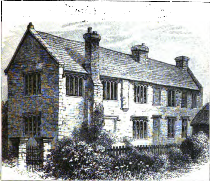
SOUTH-WEST FRONT OF ASH HOUSE, 1890.
