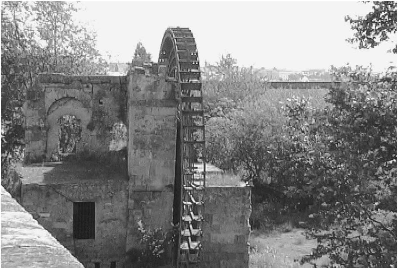
The remains of a Muslim watermill on the Guadalquivir River in Córdoba in Spain (Courtesy Edward English)
