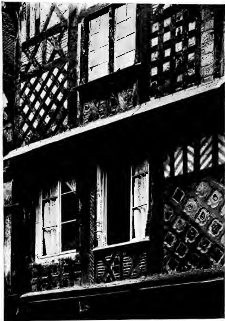
BEAUVAIS. HOUSE FRONT, c. 1550. TIMBER WORK SET WITH COLOURED POTTERY
