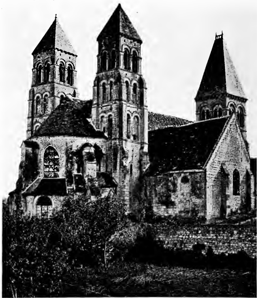
MORIENVAL ABBEY CHURCH (c. 1125) BEFORE "RESTORATION"
