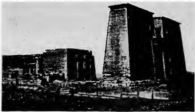
FIG. 11.—Pselkis: Temple and Pylon.
