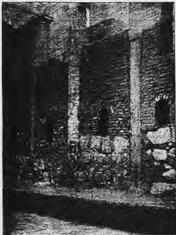
FIG. 143.—The White Monastery: Walled-in columns of nave. (Photo. by J. G. M.)
