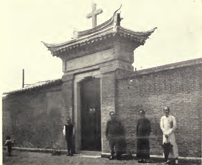
THE CREEK WHICH MAKES ST. JOHN'S UNIVERSITY CAMPUS A PENINSULA THE MAIN ENTRANCE TO THE MISSION COMPOUND, WUSIH
