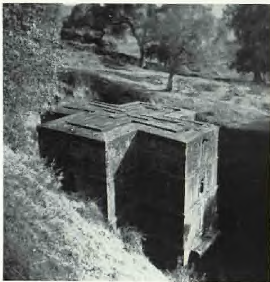
[57] Lalibela: Church of St. George, early thirteenth century. This is a good example of a rock-cut monolith, cruciform in plan, rising above a high stepped podium. According to tradition, the craftsmen who made these remarkable monuments came from Alexandria, but there are certain details which bear the indisputable hallmarks of Aksumite art. One might however detect a foreign influence in certain of the panelled ceiling designs, exact replicas of which are to be found in Central Asia, in the Hindu-Kush and Pamir regions (Photo Roger Sauter)
