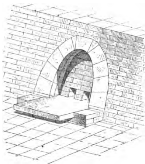
FIG. 94.—Sewer at Khorsabad, with elliptical vault ; compiled from Place.
