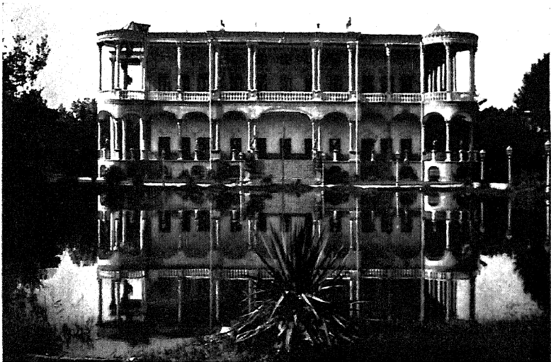
FRONT VIEW OF ATABAK PALACE TAKEN FROM ACROSS THE LAKE.
