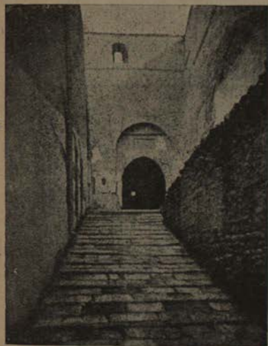
Fig. 47.—Gate of Steps in Citadel of Cairo, 1183.
