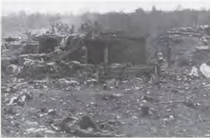
Top: Bunkers inside Camp Tong Le Chon, fabricated from reinforced steel CONEX containers, had much of their overhead timber protection and sandbagged shellburst-absorption walls blown away during the battle. Dead enemy sappers litter the ground in front of the shrapnel-riddled bunker parapets. (Author's Collection) Center: Two soldiers killed in a mutually fatal exchange of fire fell on opposite sides of an interior sandbag wall during the height of the battle for Tong Le Chon. The fallen Special Forces defender can be seen inside the walled trench, center, while his VC adversary lies at the entrance, in the left corner. (Author's Collection) Bottom: CIDG casualties are gathered by Staff Sgt. Morganfield, the Detachment A-334 medic, along the south edge of the airfield at daybreak following the battle for Camp Tong Le Chon. (Author's Collection)
