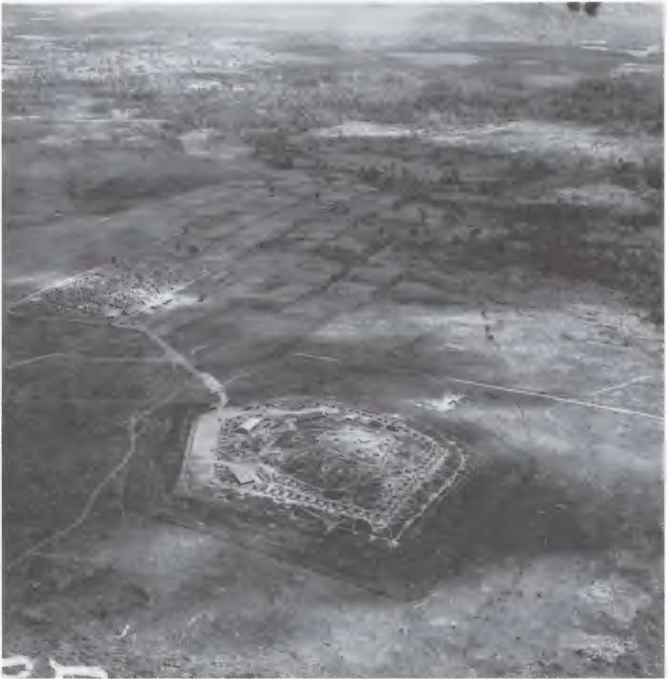
Camp Buon Ea Yang provided security along the main overland supply route to Ban Me Thuot. It was located on a 50-meter hilltop in a marshy valley about 15 miles from the Vietnamese coast. When completed, three double-apron barbed wire fences and a trench with firing bays and nine machine gun bunkers encircled the camp. The bunkers were situated at each of the camp's five corners and at the center of each trench line. The camp contained two light howitzers that covered the main avenue of approach from the southwest, six light mortar positions, ■ main barracks building surrounded by a log parapet with another machine gun position, and a zigzag trench leading to the upper trench system with four heavy mortars and the main bunker. (Author's Collection)
