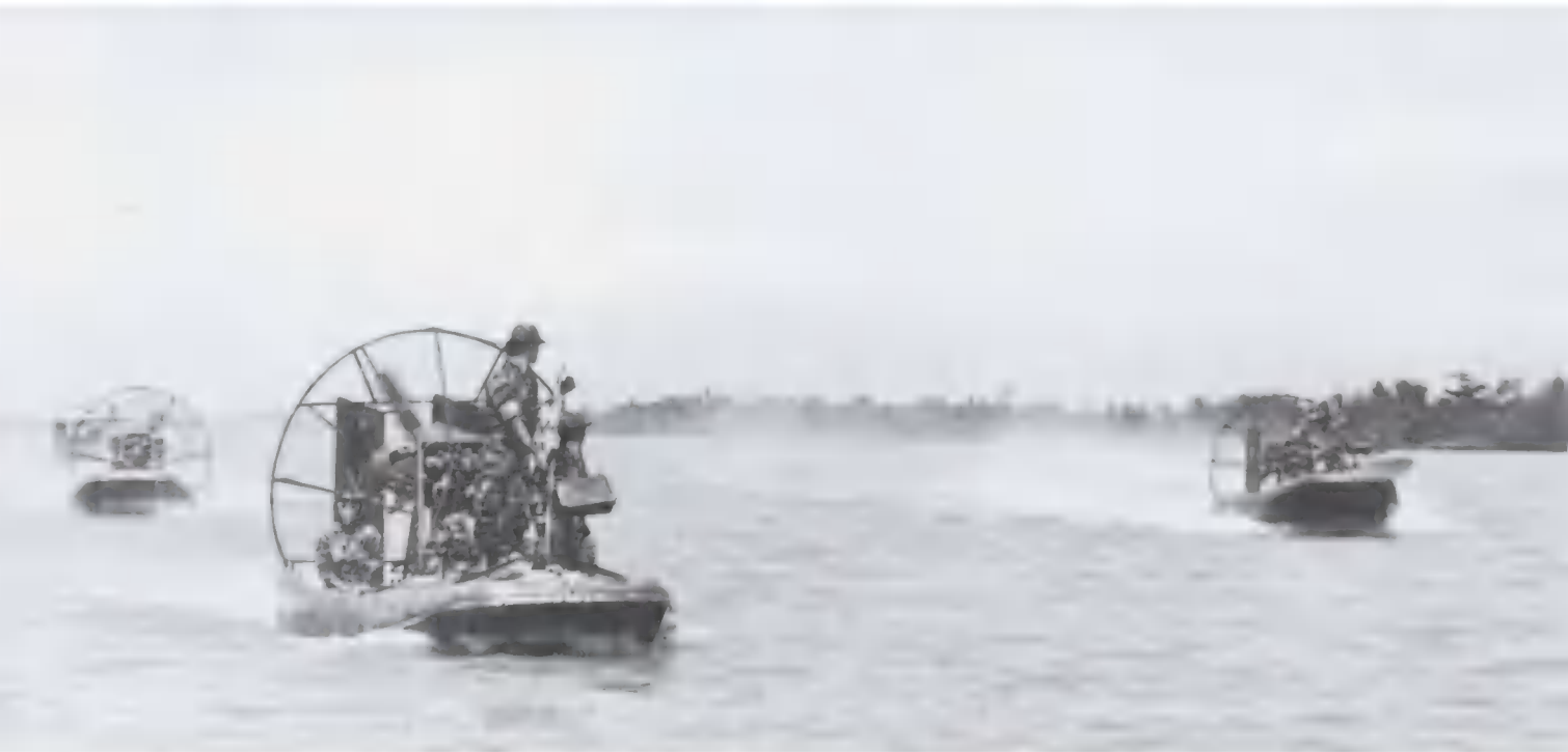
Top left: Airboats from Camp Thuong Thoi in the open marshes of the Plain of Reeds near Cambodia during September 1967. The highly maneuverable boats were powered by 180-horsepower Lycoming aircraft engines. ( Author's Collection ) Top right: The flexibility of airboat operations is demonstrated as CH-47 Chinooks airlift two sections of IV CTZ Mike Force airboats from Don Phuc to the Seven Mountains region during November 1966. ( George Marecek ) Center: An airboat formation of Special Forces Company D travels along the Mekong River near the Cambodian border in late 1966. The Hurricane Company Aircats were capable of going 38 miles per hour when carrying 300 pounds. ( 5th SFG PIO ) Bottom: Special Forces monitoring of the waterways included using Vietnamese officials aboard airboats, such as this national policeman checking the identity papers of a fishing couple in the Delta during September 1970. ( Ensign/USA )
