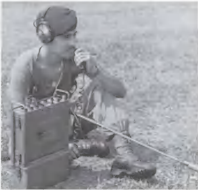
Top: The Air Force multichannel survival radio was often carried by Special Forces long-range patrols to contact reconnaissance aircraft, provide spot reports, and relay emergency-extraction instructions. (USAF) Center: The PRC-74 single-sideband radio was used by Special Forces patrols operating beyond the range of portable radios issued to regular troops. In October 1966 the nickel-cadmium battery case was introduced by Special Forces to increase the radio's utility. (Richard Nieland/USA) Bottom left: Introduced in 1968, the Beacon System used by Special Forces long-range patrols determined a patrol's position for precise fire support. The Patrol Station Assembly, shown here, used a low radar frequency to penetrate through heavy foliage and communicate with two other base stations to determine ranging. (DOD) Bottom right: Communications chiefs of the 5th Special Forces Group with signal officer Maj. Bowles at Nha Trang in February 1970. These high-ranking sergeants were responsible for the vital field-communications link between far-flung elements of the Special Forces empire in Vietnam. (5th SFG PIO)
