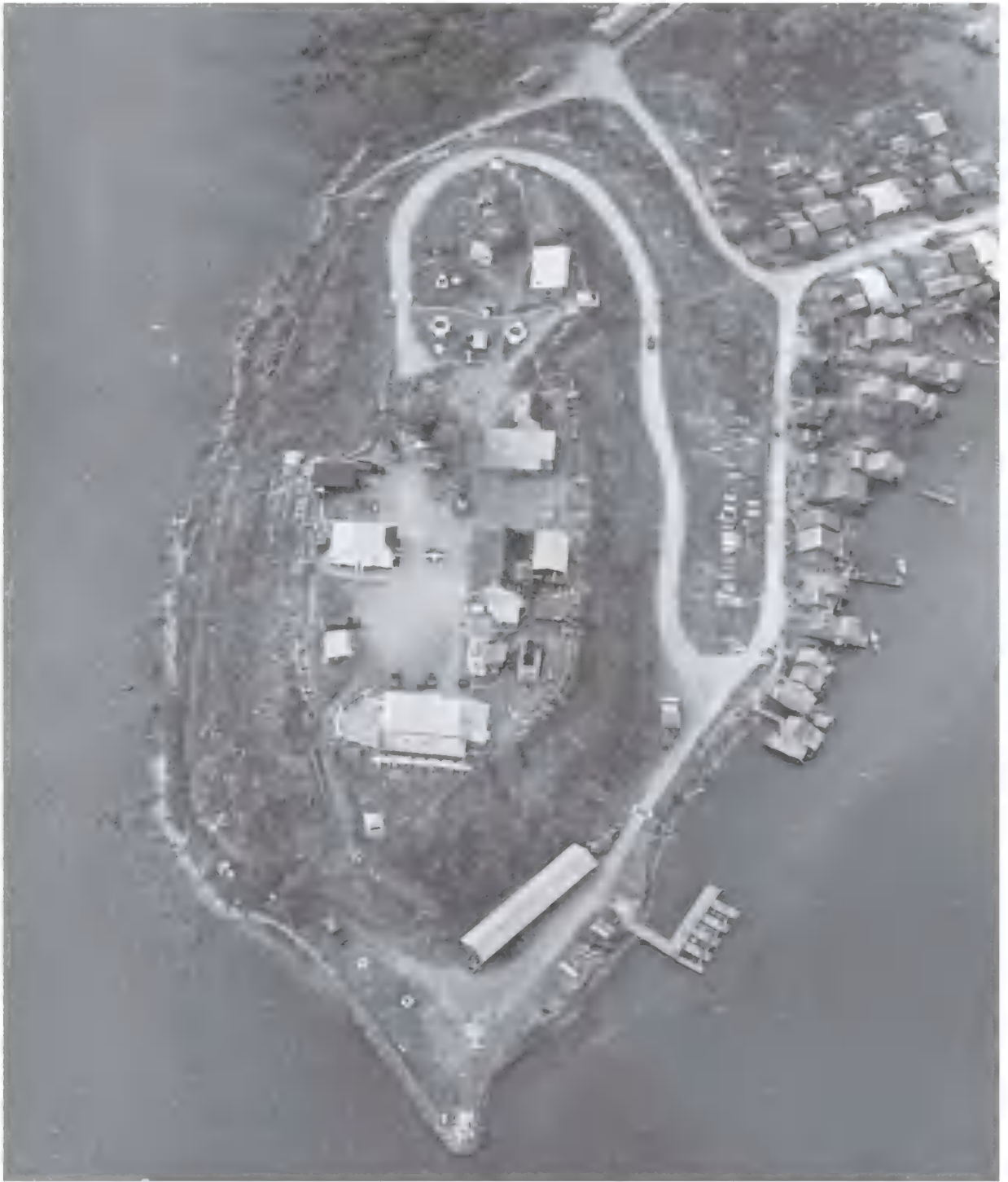
Camp Ha Tien on the South China Sea was the southern anchor of the projected Special Forces border line. It was situated in the extreme southwestern tip of Vietnam's Mekong Delta, adjacent to Cambodia. Ringed by a hilltop trench line and several mortars that offered good protection for this stage of the war, the camp served as a training base for Vietnamese border-surveillance leaders. (Author's Collection)
