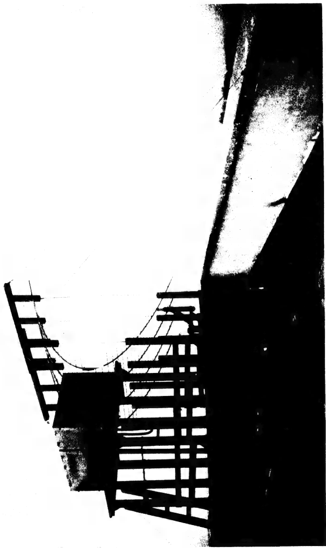
Marconi ultra-short wave reflector or radio "searchlight" on top of the Vatican station "beams" a 56-centimeter wave across a distance of about fifteen miles.
