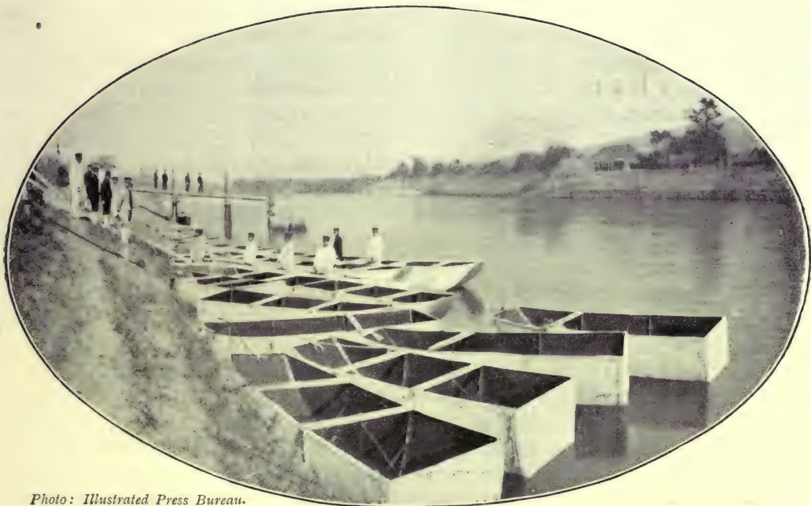
JAPANESE PIONEERS BUILDING A BRIDGE: SHOWING FORM OF PONTOONS.
