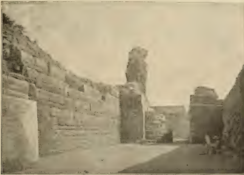
FIG. 335. BCA . I. p. 29, f. 23. Greek walls at Chersonese looking SE. from near e towards Dd . Seven courses of first period, four of second with round tower D . Upper work and square towers Dd , Roman.
