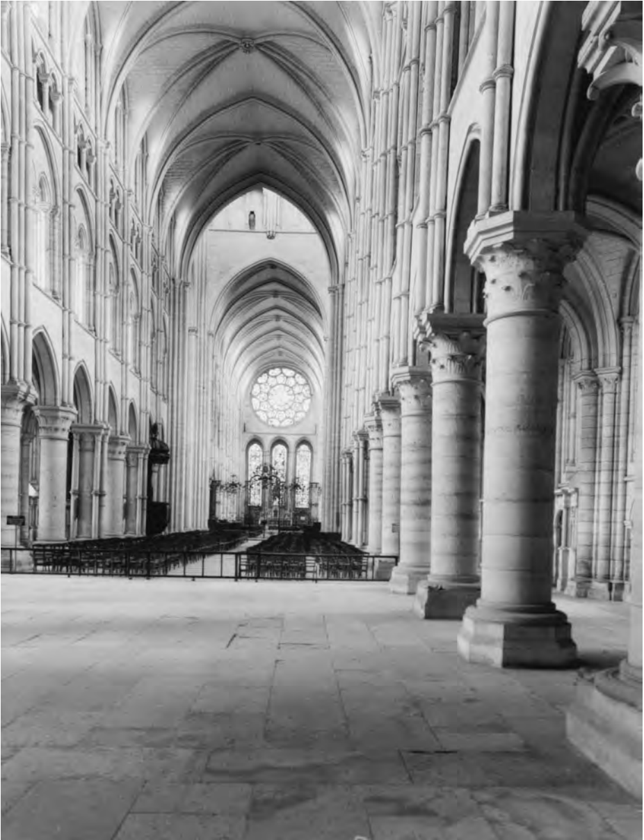
21. Laon cathedral, nave interior, last quarter of the twelfth century.
