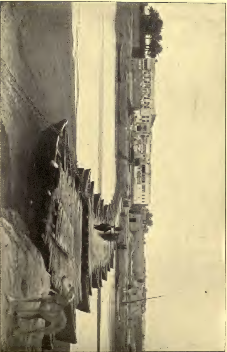
BRIDGE OF BOATS ACROSS THE LOWER TIGRIS. Over the boats, which are of the very simplest construction, are laid poles, and over them rushes, the whole making a somewhat uncertain platform. In the foreground is a greyhound, such as are rather common in Eastern Turkey.
