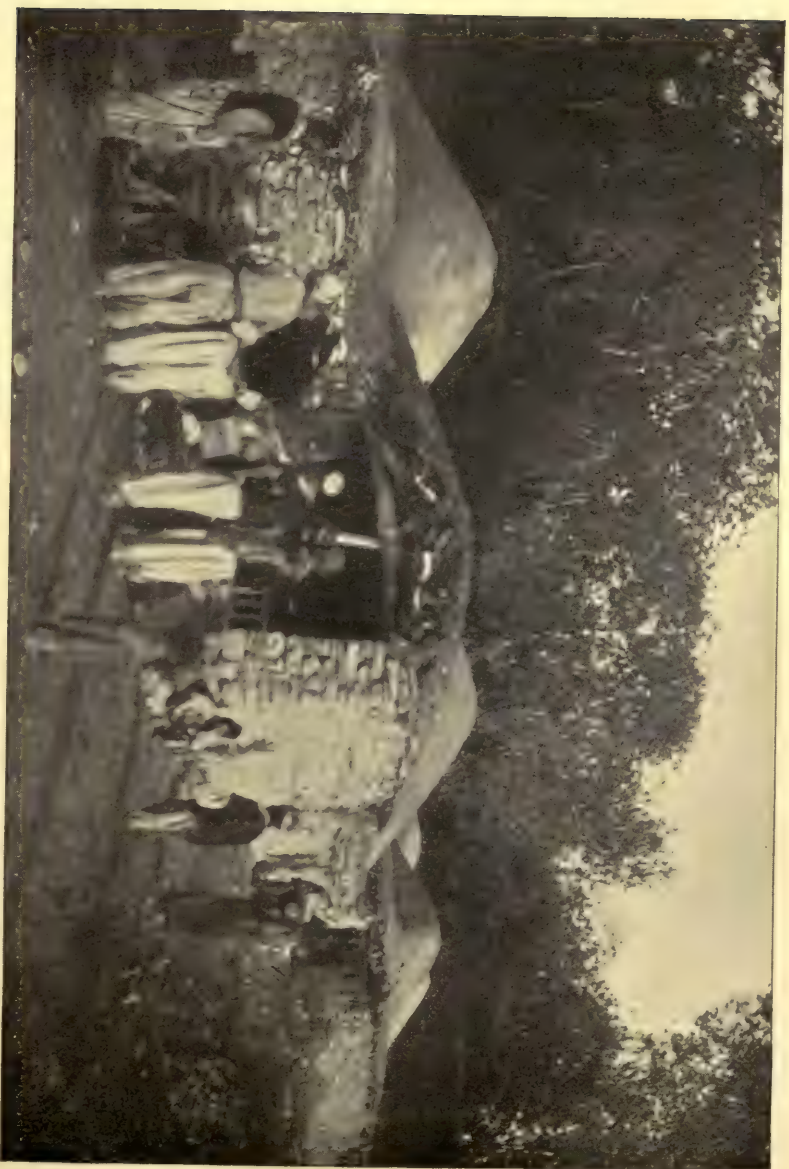
KURDISH MOUNTAIN VILLAGE. A typical scene in the mountains. There is a group of houses mostly connected by passages half under ground. The walls are of rough stone. The roof is formed, as seen, by rough beams, over which branches are stretched and earth over them, sometimes formed into a dome, in which there is a hole serving as window and chimney.
