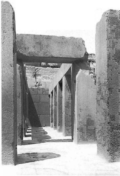
(Above) The ancient Egyptians' complete mastery of working hardstone is well exemplified in the interior construction of Khafre's valley temple, where great blocks of granite may be seen with most strange, almost tenon-like joints, often turning corners instead of being cut to butt ends.
