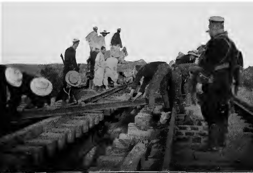
CHARRED SLEEPERS AND WARPED RAILS ON THE LINE OUTSIDE TIENTSIN.
