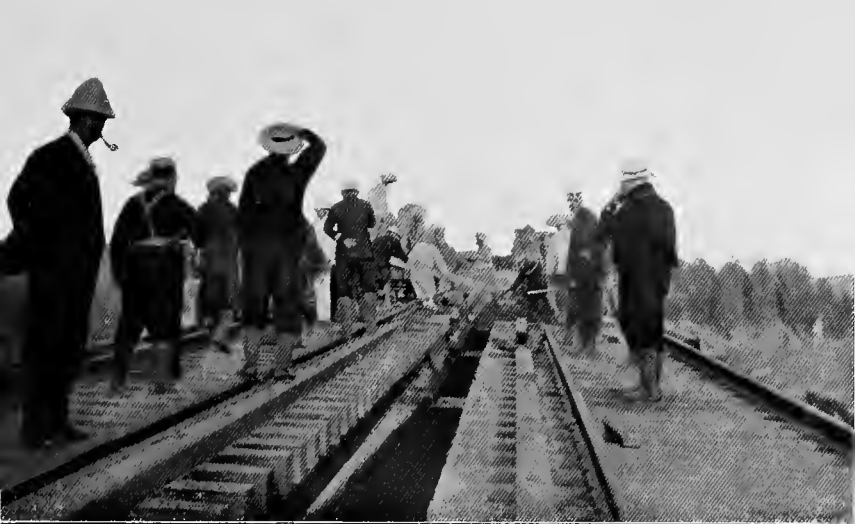
REPAIRING THE LINE OUTSIDE TIENTSIN.
